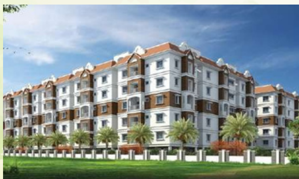
CASCADE GREENS Kompally
